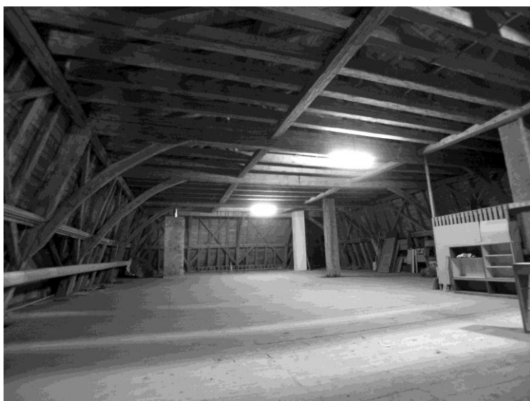
La charpente – Photo Raymond Gruaz
